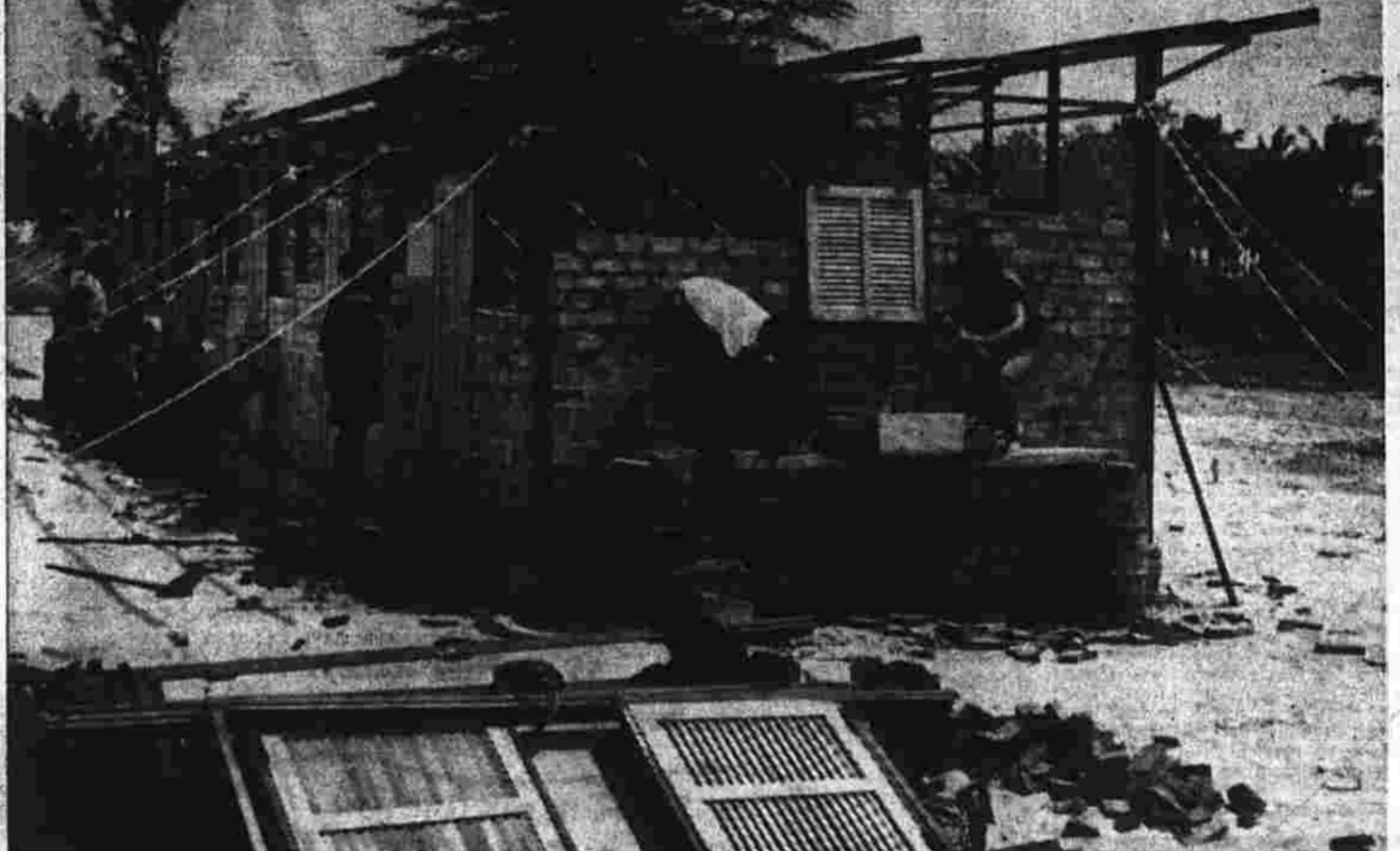
Crossroaders and Senegalese laying bricks at schoolhouse construction reaches halfway mark.
